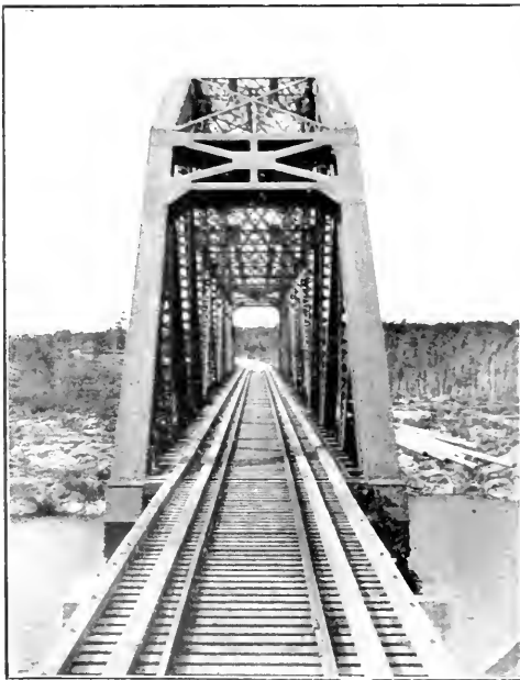
THE BRIDGE OVER THE PICKEREL RIVER
